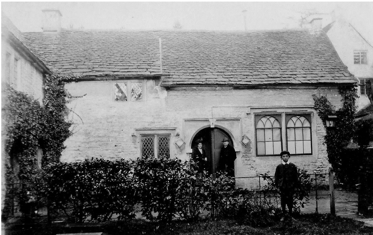
Figure 1: Undated (early twentieth century?) photograph showing Georgian Gothic glazing and panelled doors (photo courtesy of local meeting)
